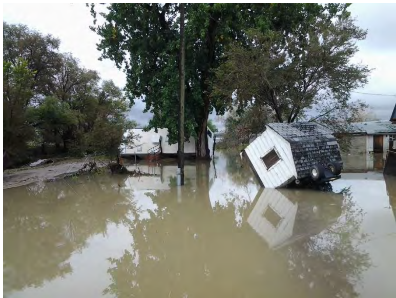
FIGURE 31. DAMAGES FROM 2013 FLOOD EVENT
