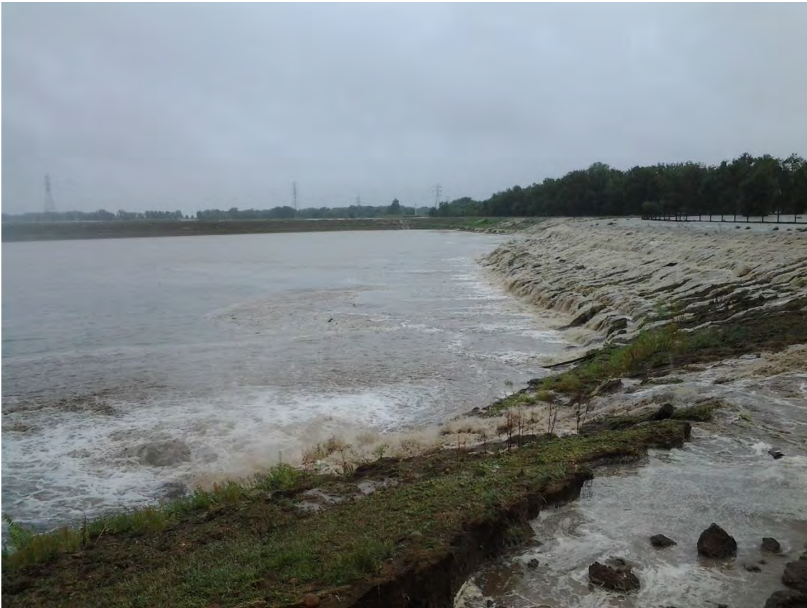
FIGURE 45. PLATTE RIVER BREACH AT ARVADA CELL (2013 FLOOD)
