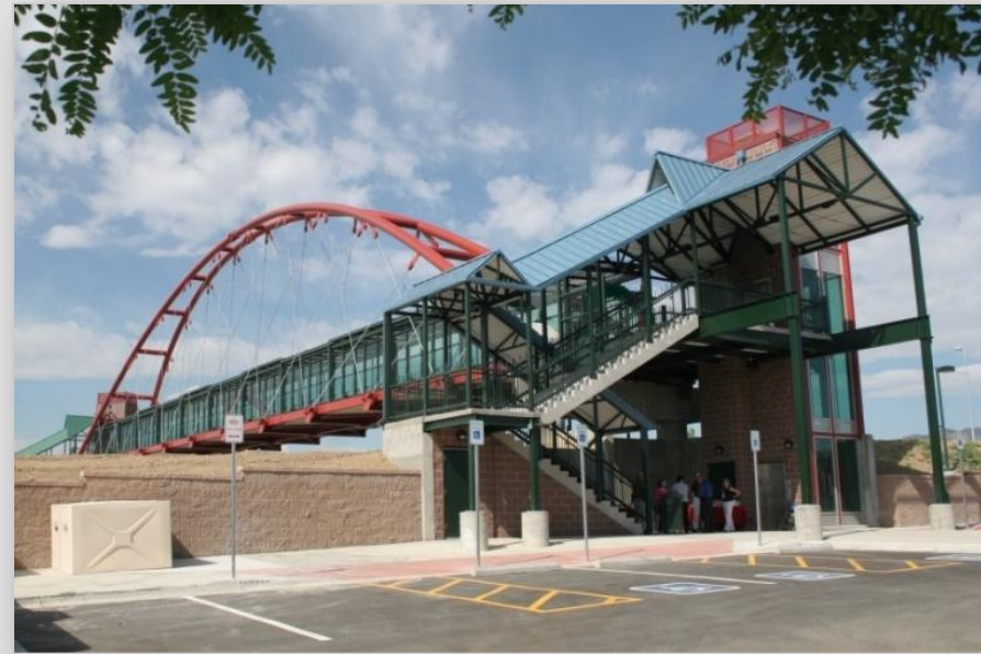
US 36/McCaslin Pedestrian Bridge
