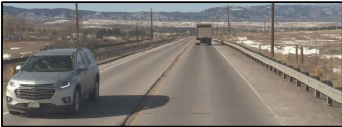
Figure 1: US-85 MP 185.60-189.55 Typical View
