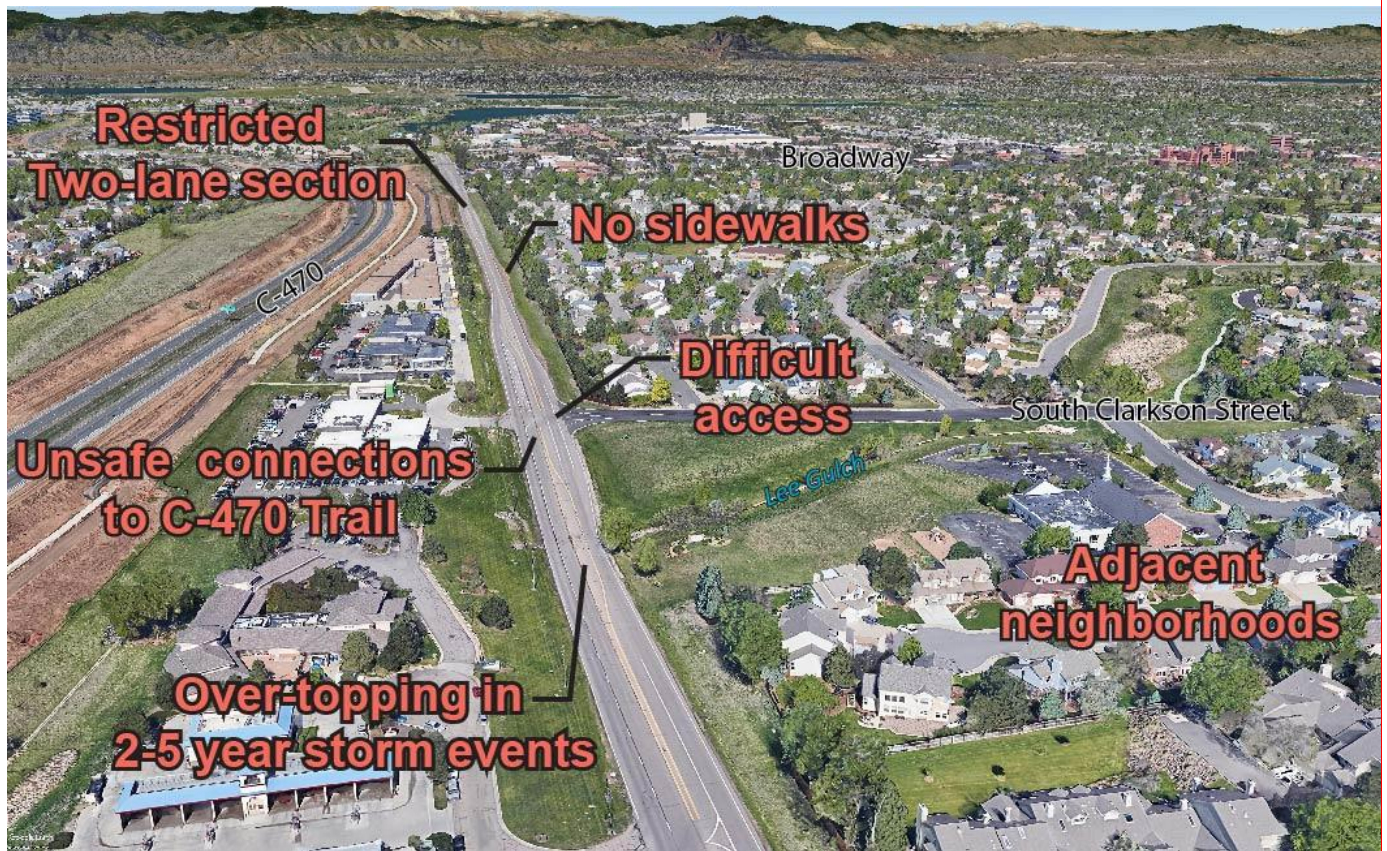
County Line Road - Existing Conditions
