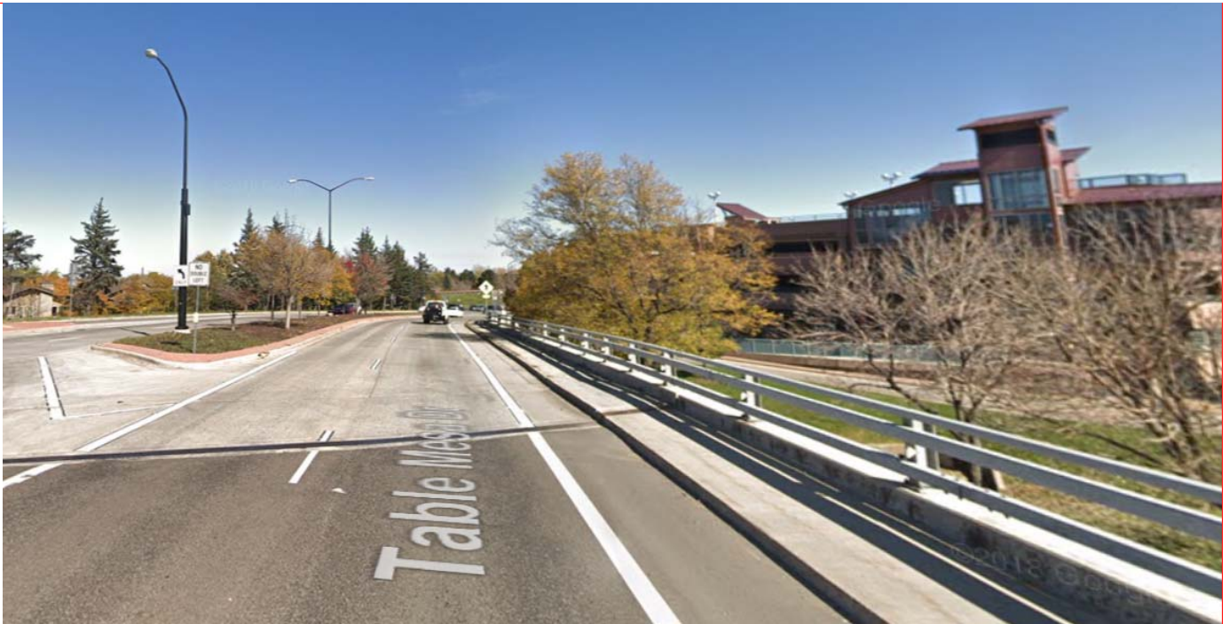
View of the south side of Table Mesa Drive looking east at Table Mesa park-n-Ride
