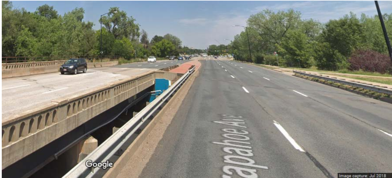
From Arapahoe Avenue bridge over Boulder Creek looking east.
