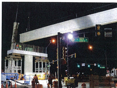
Construction crews set girders on the Illiff Avenue light rail bridge.
