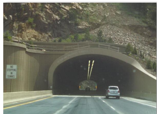
I-70 Eastbound Twin Tunnels
