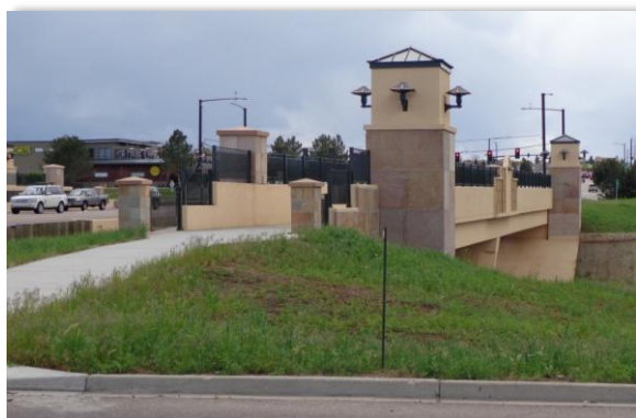
Quebec Avenue Overpass of C-470
