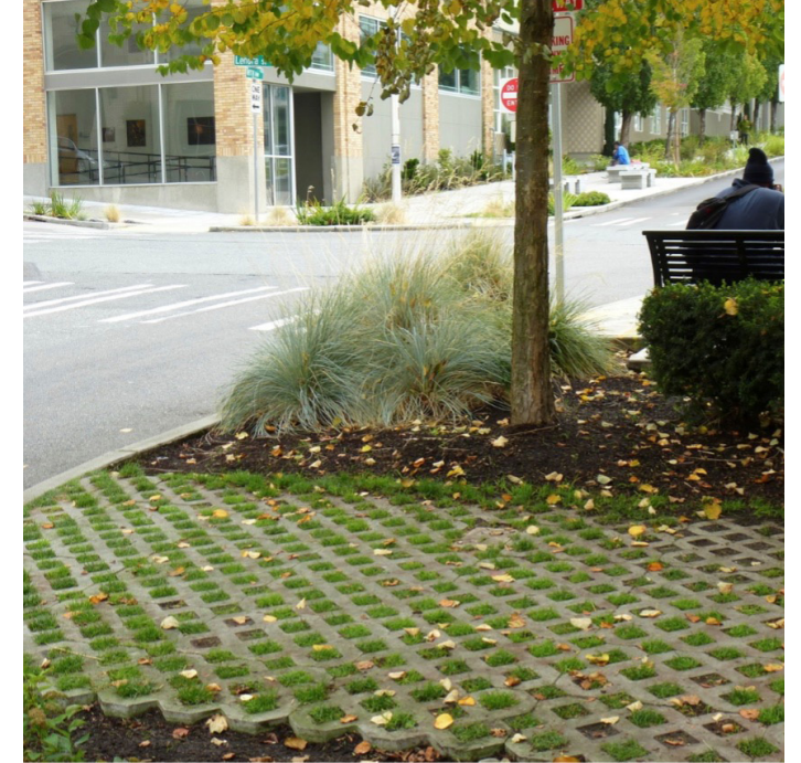
Consider different pavement types, such as permeable pavement, in appropriate locations to provide green infrastructure.
