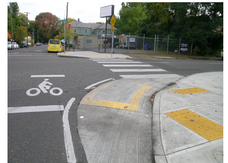
Mountable truck aprons slow the most common passenger vehicles while still allowing larger vehicles to make the turn. Rapid implementation versions can also be installed using rubber speed humps.
