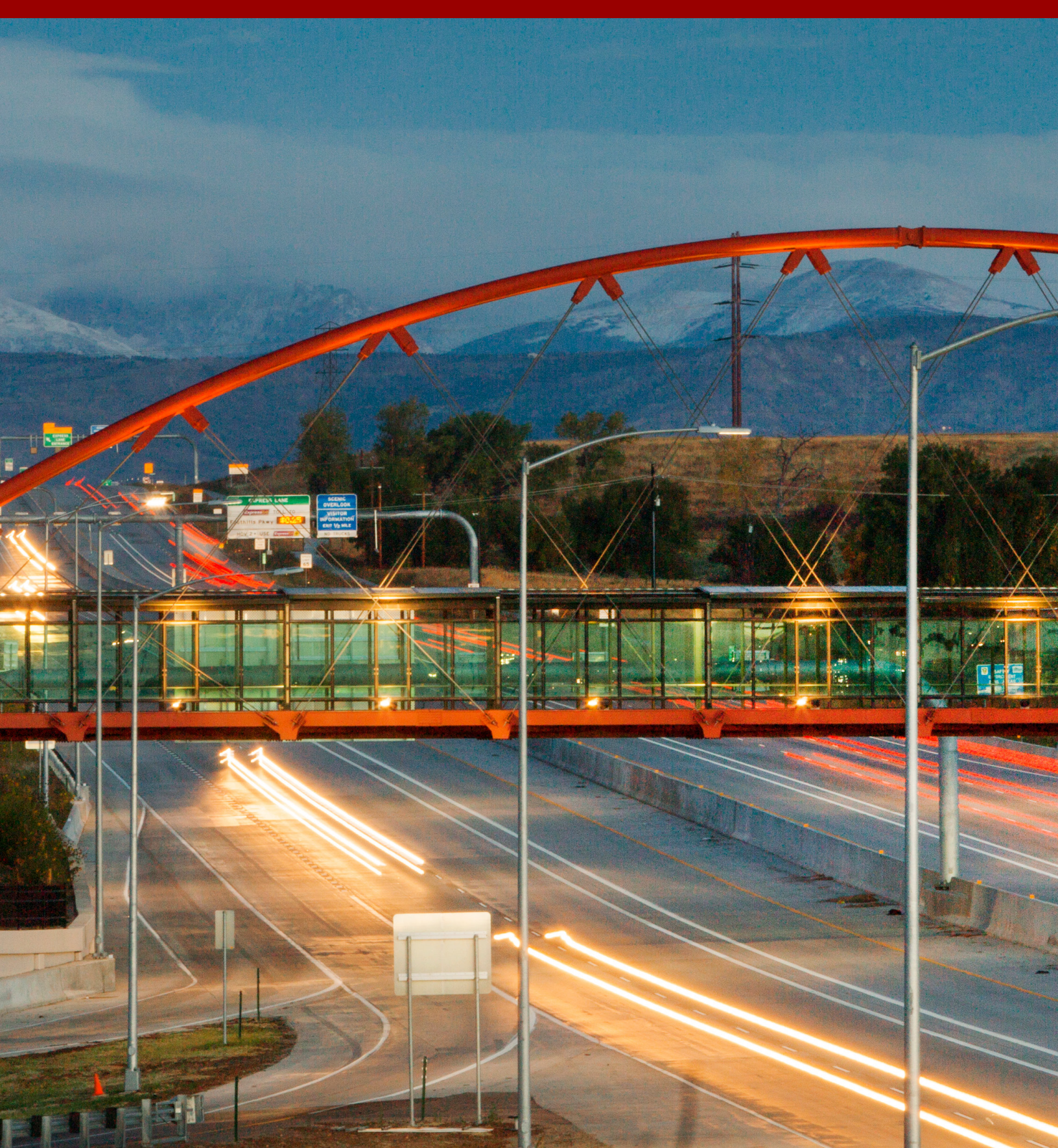
U.S. Route 36 is a busy highway that connects Denver and Boulder. Photo by Ground Floor Media, courtesy of CDOT.
