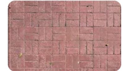
**Bricks and stone pavers** can be confusing, as blind users may not know if their use is intended as tactile communication or is purely aesthetic. Designers should be judicious about use of pavers or stamped concrete surfaces.
