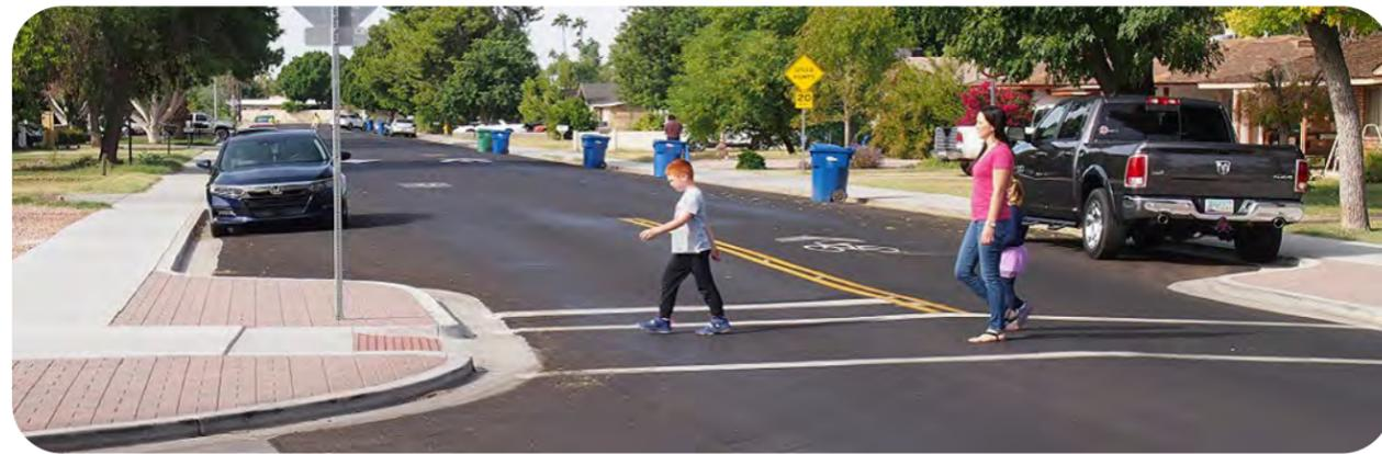
Figure 22 Curb extension (Source: Alta Planning + Design)
