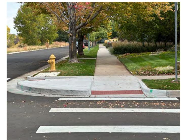
Figure 17 Example of an accessible curb ramp.
