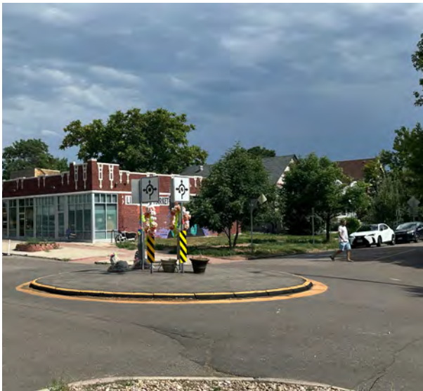
Mini traffic circles and traffic diverters
