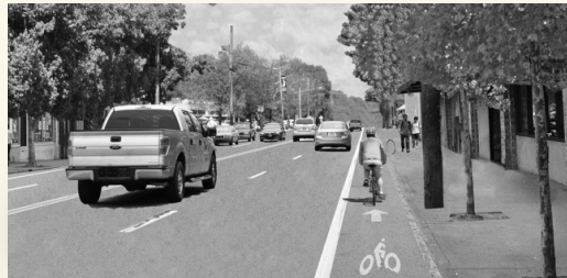
Bicycle lane on a four-lane roadway.
