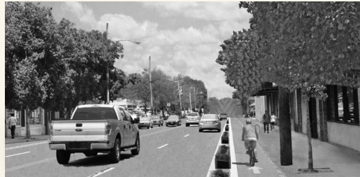
Separated bike lane on a four-lane roadway.
