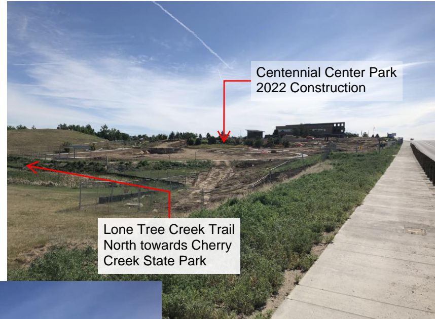
Figure 3 - Arapahoe Road Underpass Project Location (Facing North & East)
