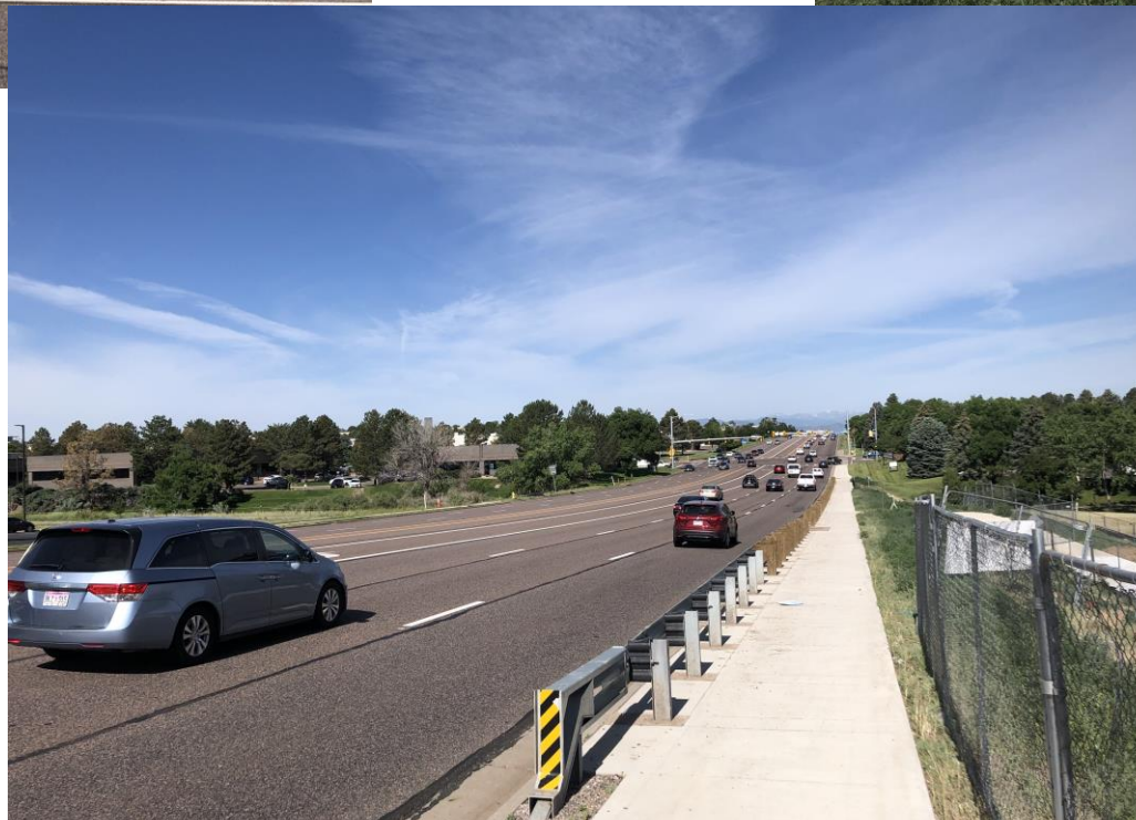
Figure 2 - Arapahoe Road Underpass Project Location (Facing West)
