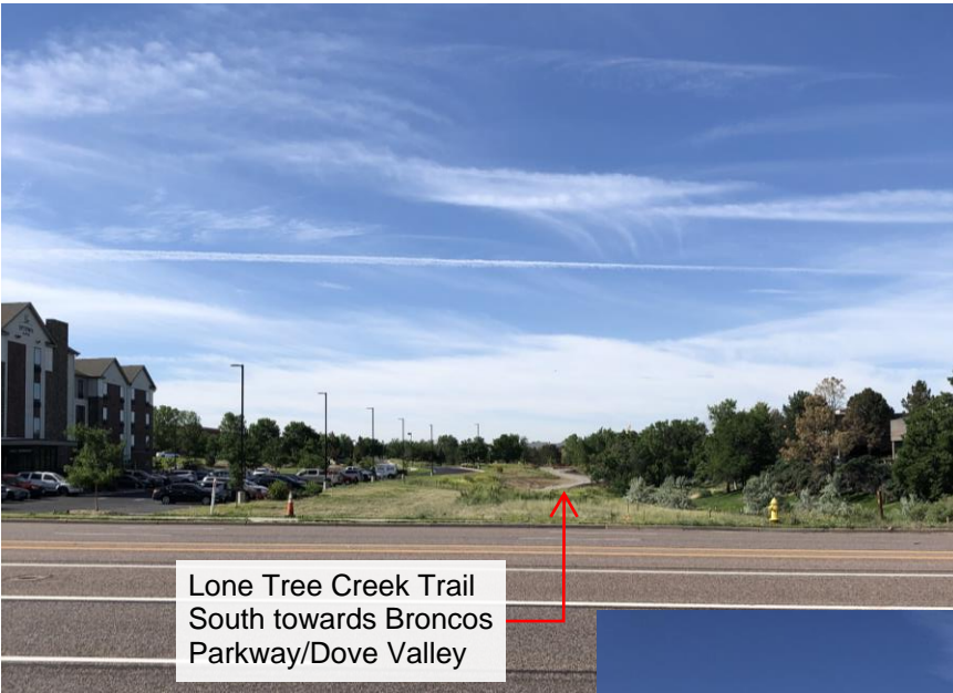
Figure 1 – Arapahoe Road Underpass Project Location (Facing South)
