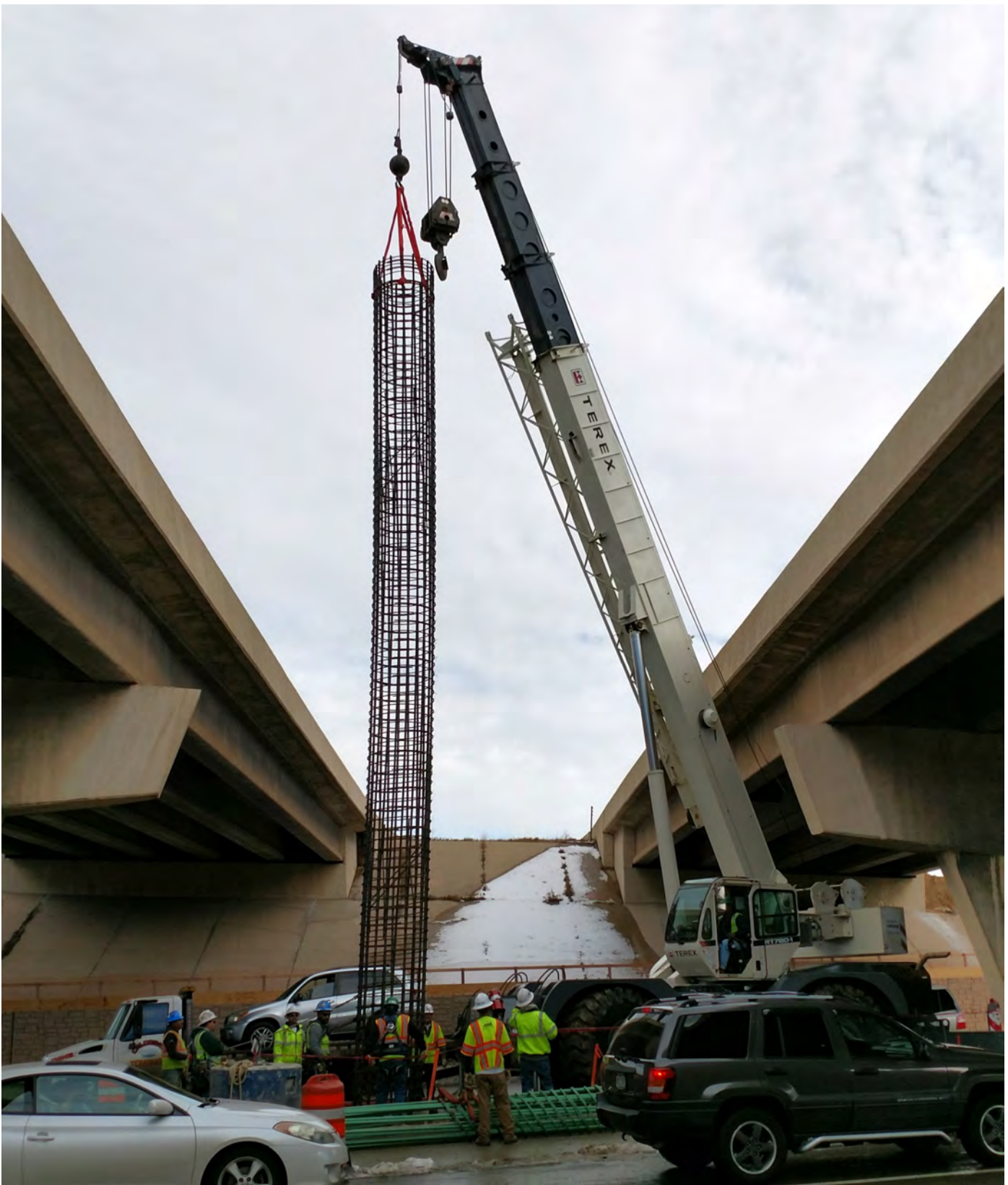
The Colorado Department of Transportation conducts foundation work at Broadway for bridge widening as part of the C-470 Express Lanes project. More than 100,000 motorists daily use the section of C-470 between Interstate 25 and Wadsworth Boulevard.
